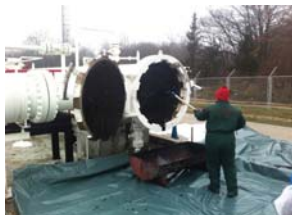
Removal of paraffin and sludge at the cleaning pig exit of a large diameter crude oil transport pipeline.
